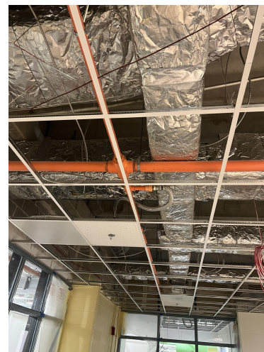
Installing ceiling grid and fire sprinkler rough-in on level 2.
