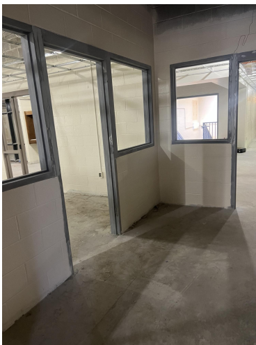
Window frames installation and painting in the security vestibule on level 2.
