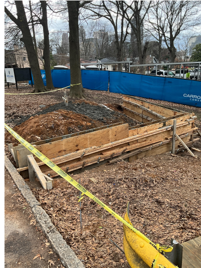
Installing the retaining wall and pad for the transformer
